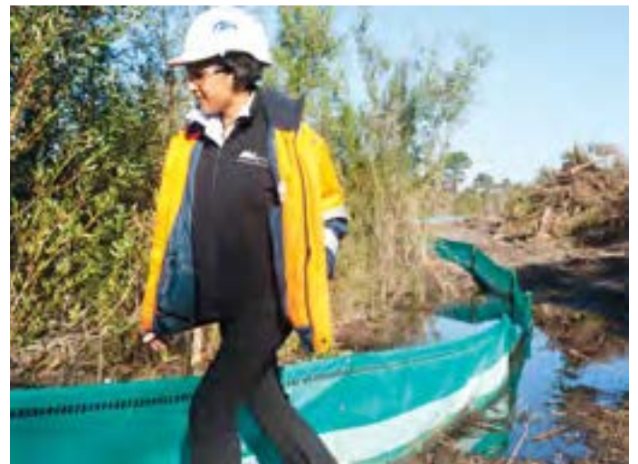
Sediment fencing filters clean water into existing waterways.
