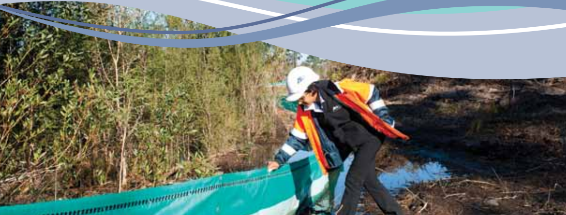
Sediment controls in place to protect Dwarf Galaxias habitat.
