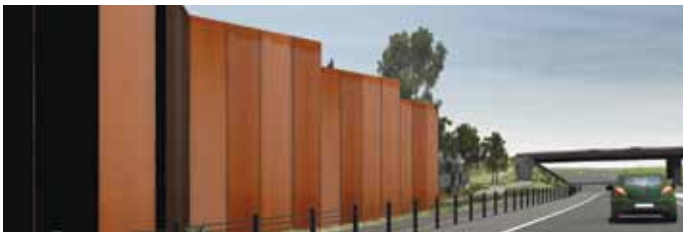
Figure 1 : Oxidised noise wall.
