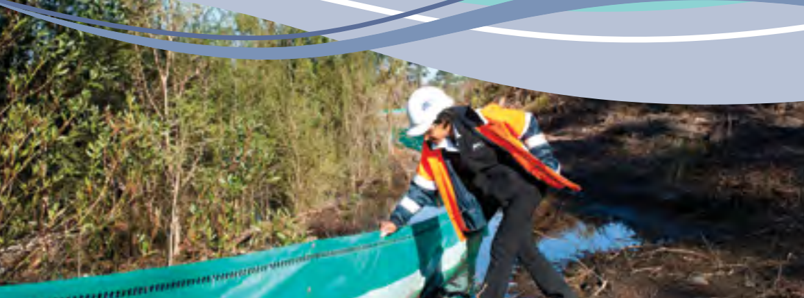
Sediment controls in place to protect Dwarf Galaxias habitat.
