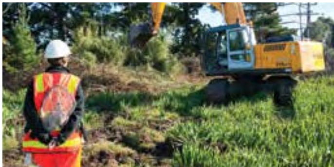
An environmental rescue officer monitoring vegetation clearing.
