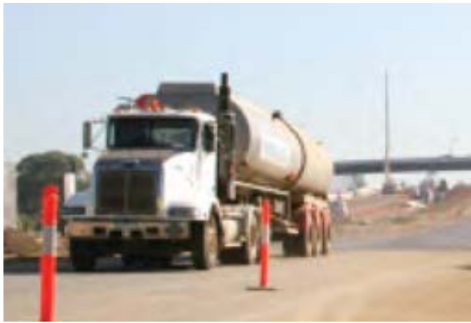
Water Trucks are put in place to control dust.
